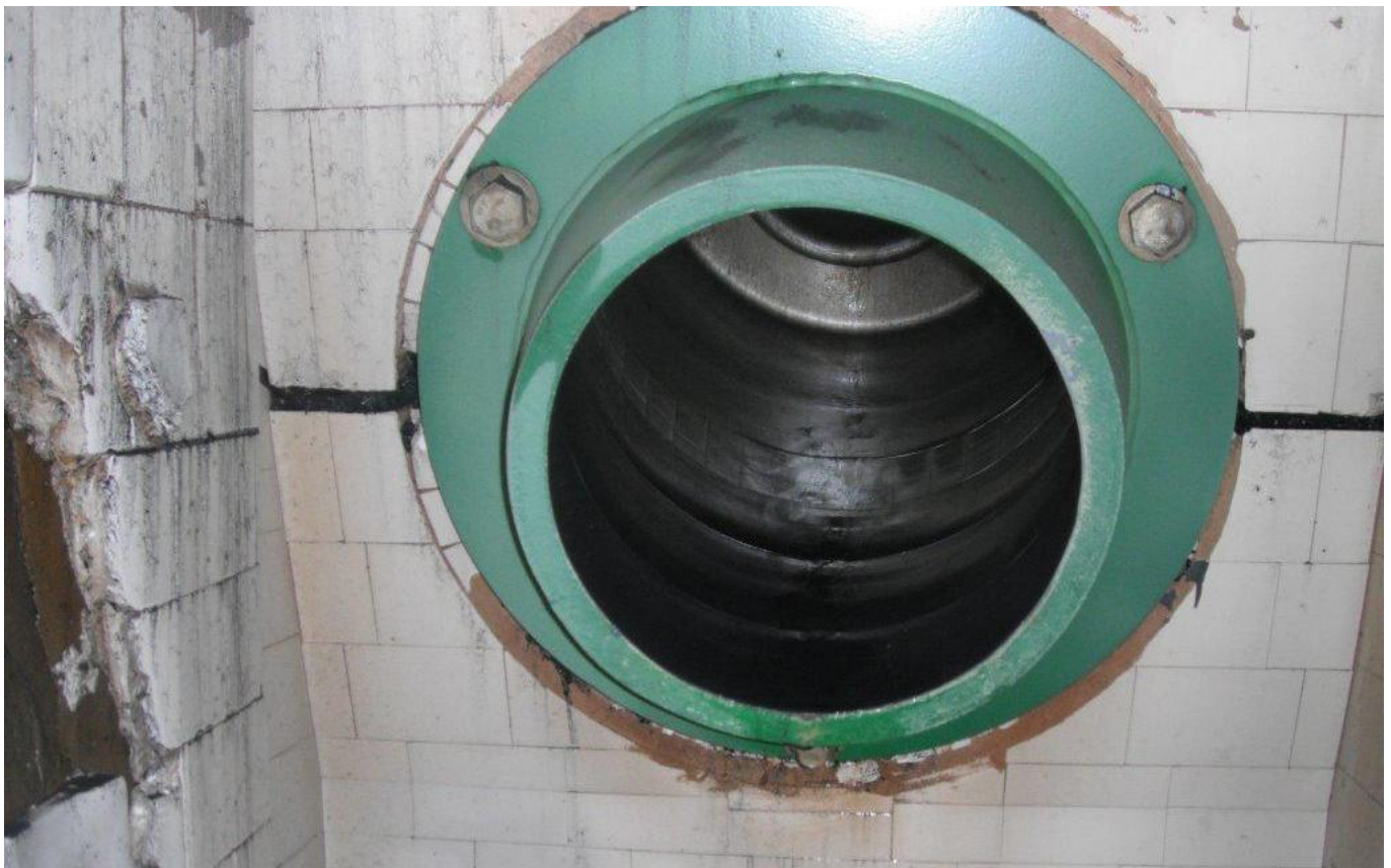
SiTech Spigot and Lower Cone
