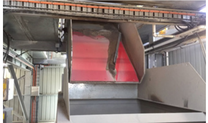
HMA Uretech sheet fitted to the right hand side hopper.
