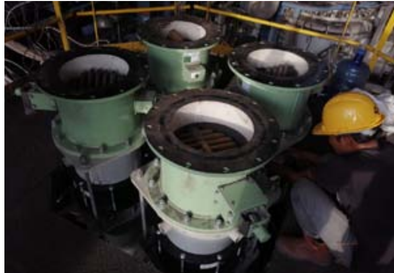
CoalFlo® dampers being installed
