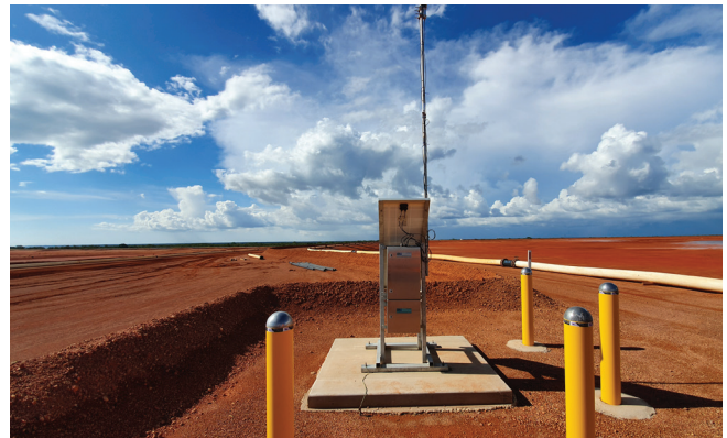
On-site photo of base station (RSTAR 'Hub'), housed in a protective enclosure and shown with the installed omni antenna and solar panel.
