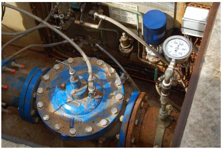
HMA successfully trial state of art motorised pressure reducing control pilot in utilities system
