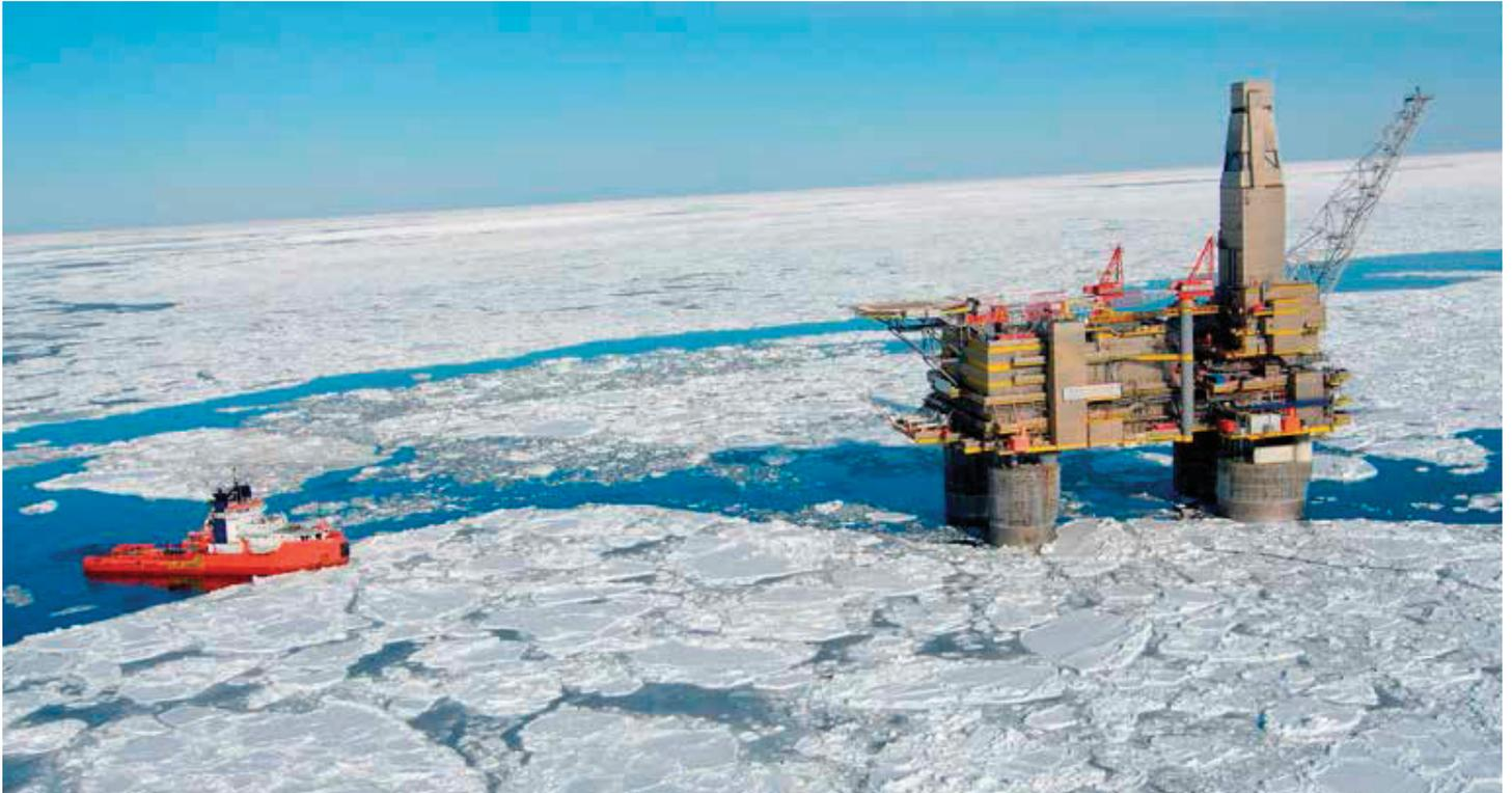
Above: Arctic gas-producing regions, which see temperatures as low as  $-60$  degrees C ( $-76$  degrees F) and can be ice-bound for seven to nine months during the year, are isolated from oil and gas infrastructure and therefore demand equipment that operates reliably without human control.
