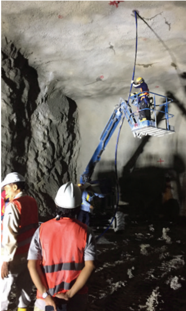
Figure 2 – MPBX installation
