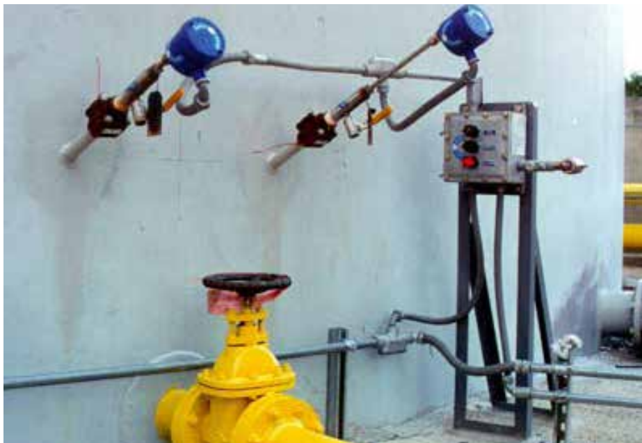
Agar ID System 1 & 2 Tank Installation
